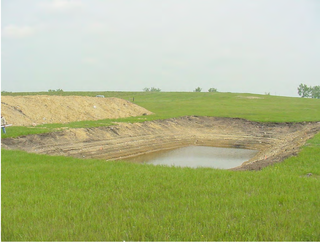
Figure 7. New Stock Pond Installed on Expired CRP Field.
