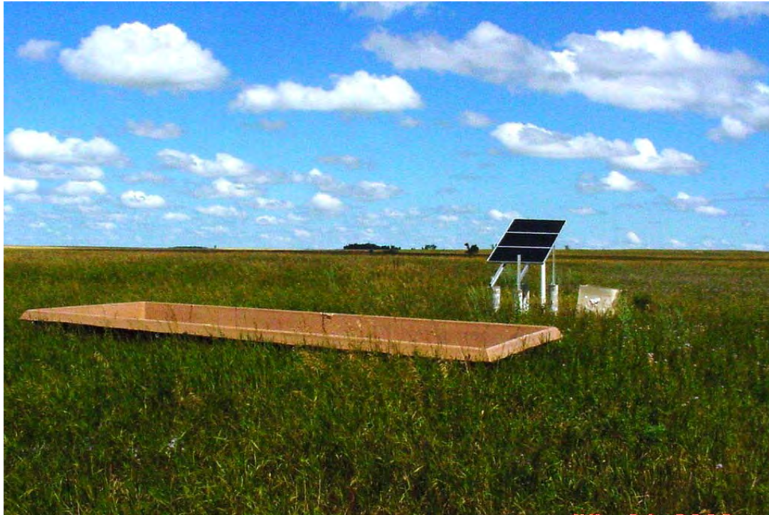
Figure 5. Solar Powered Well and Stock Watering Tank.
