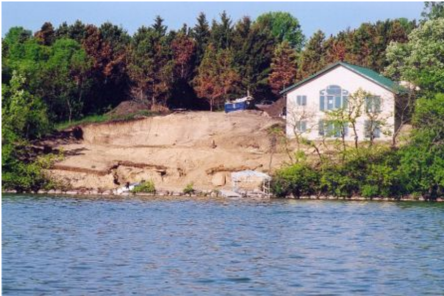
Figure 20. Shoreline development along Pickerel Lake (note failure of hay bales to stop runoff from site)
