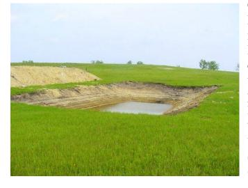
Cost share is available for new stock ponds. Ponds cannot be placed in creek bottoms and must be fenced on a minimum of three sides. It is highly recommended producers completely exclude livestock from ponds and utilize nose or solar pumps and stock tanks to pump and store water from the pond for livestock watering. These practices prolong the ponds life and will improve a ponds water quality and general livestock health. Stock ponds typically cost \$2,500 to \$3,000.00 to construct.
