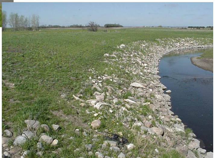
Restored stream bank after reshaping and placement of rock rip rap
